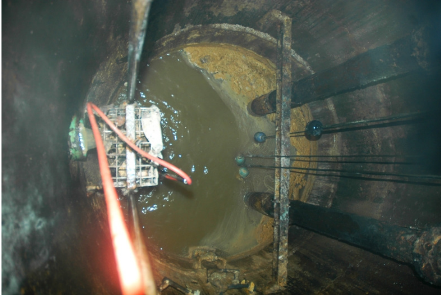
Figure 4. Lift Station after VaporX Treatment
